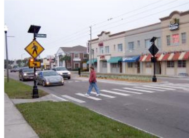
The image above displays a zebra or ladder-style crosswalk that is elevated to slow traffic. Textured and colored bricks contrast with pavement to call attention to the crosswalk (see "special paving" for more information on colored pavement). A bulbout on the right-hand side extends the sidewalk and increases safety by shortening the crossing distance and moving the pedestrian waiting area into drivers' line of sight, as opposed to behind parked cars. (Photo credit: www.pedbikeimages.org / Michael Frederick)
